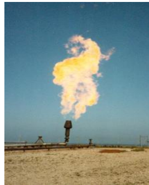
Figure 2. An operating Coanda flare.
